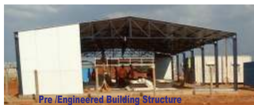
Pre /Engineered Building Structure
